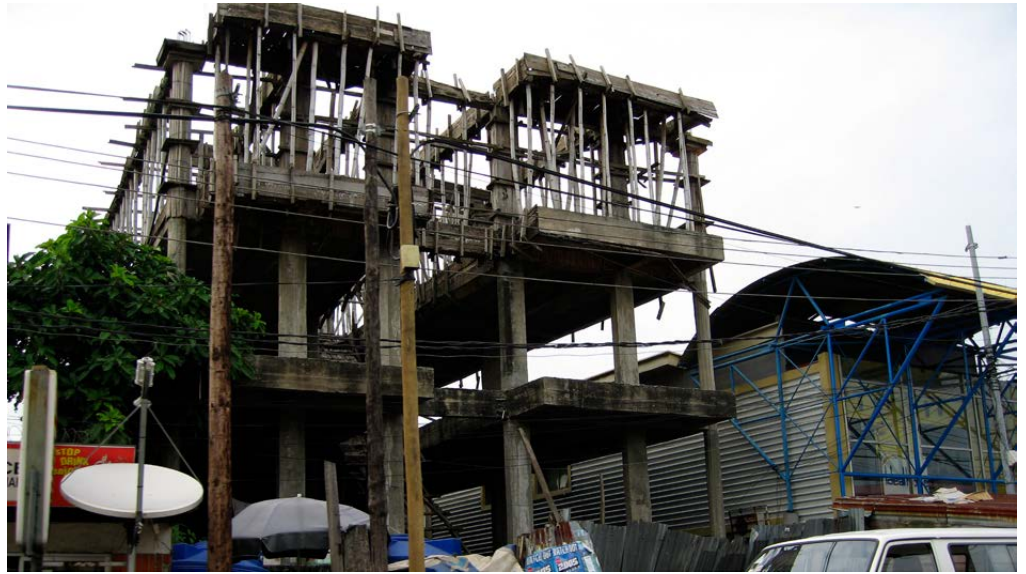
A building under construction in Lagos, Nigeria.
